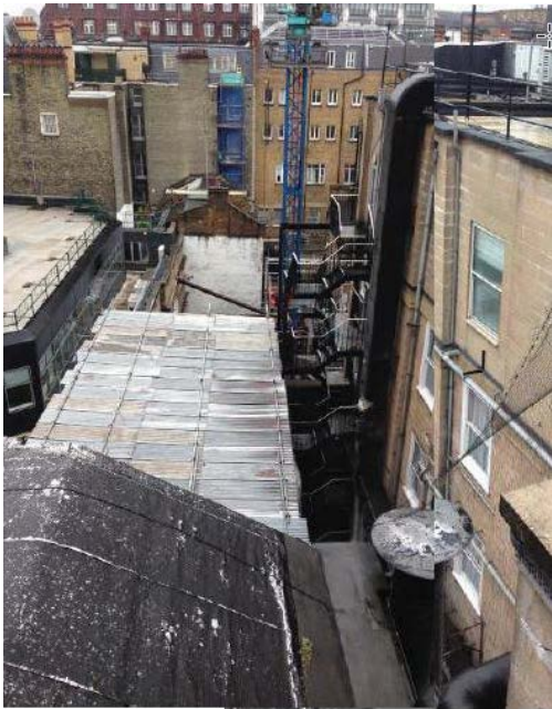
View over squash wing ( pre-construction of 3 Down Street Mews)
