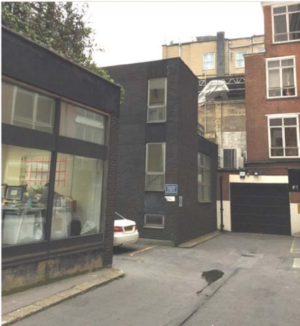
Existing view from Grantham Place
